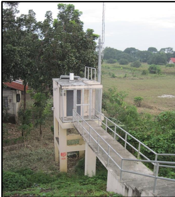
Figure 4. A photo of the new telemetered water level station.
