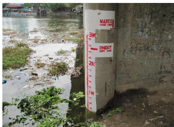
The staff gauge (above) at Bagbag River in Caniogan, Calumpit has event flood markers painted to enhance community awareness. A joint undertaking of the PRFFWC and PDRRMO-Bulacan in line with the latter's community-based flood mitigation and management program for the Province of Bulacan. (April 2010)
