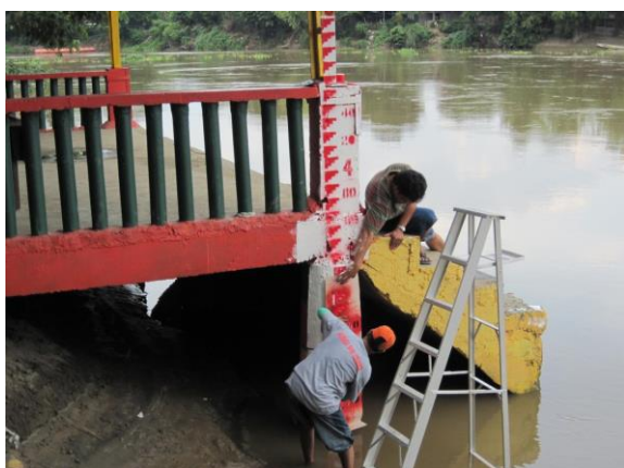
Above picture shows PRFFWC personnel painting a staff gauge at a boat pier landing in Apalit, Pampanga. The said gauge can be seen atop the NLEX bridge along Pampanga River in Apalit plying the northbound side at upstream, right bank of the river. (February 2010)
