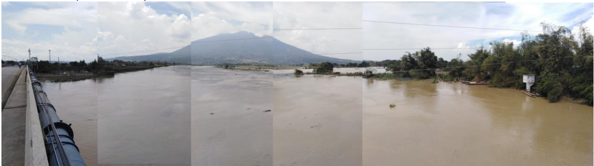
Upstream view of the Pampanga River at Arayat station just after the passage of Super Typhoon “KARDING” over the PRB; the river view shows an estimated staff gage reading of 7.98 meters (above ALARM WL) at that time of the photo, 1100H, 26 Sept. 2022.
