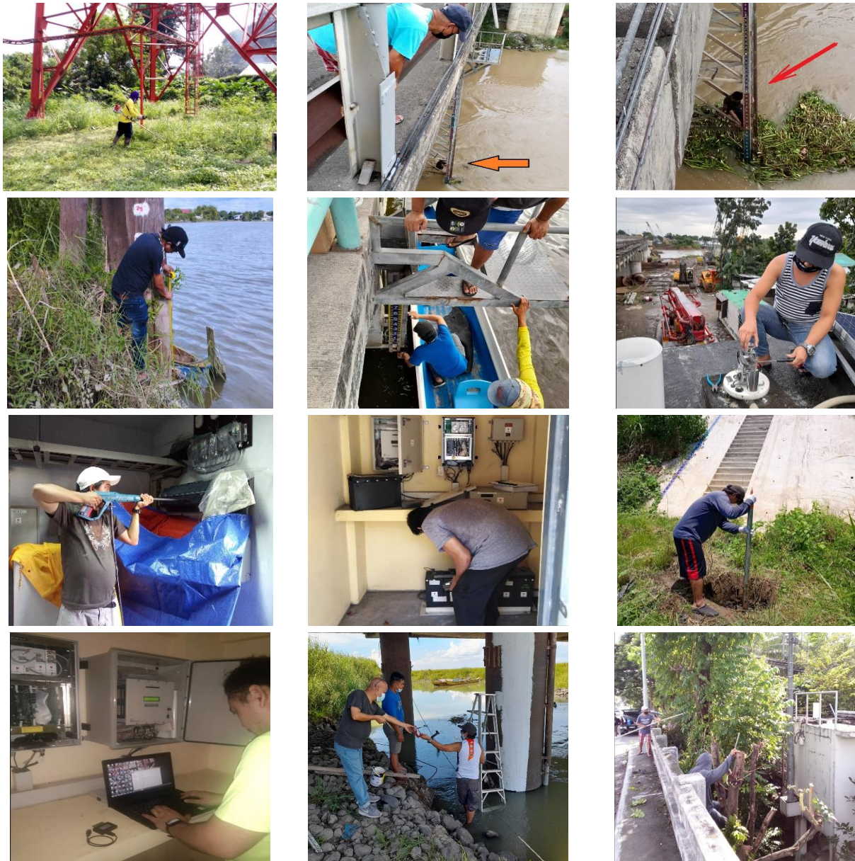
Above pictures shows some of the various activities being carried-out during quarterly maintenance of the technician group of PRBFFWC. Maintenance activities includes, among others, cleaning of station surrounding (top left pic & bottom row right); cleaning and installation of staff gages (top middle and right, 2 nd row middle & bottom middle); cleaning of instrument (2 nd row right); cleaning of air conditioning units (3 rd row left); declogging / desilting of sensor pipes (3 rd row right); backup of logger data and checking of telemetry power (bottom left & 3 rd row middle, respectively)
