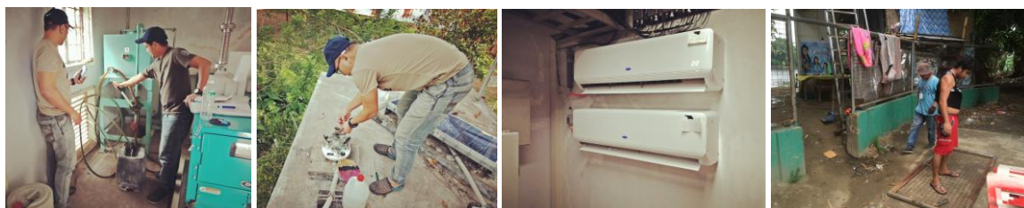
(Above pictures, L to R) PRFFWC personnel filling-up the diesel tank of the San Rafael Repeater's generator set; Cleaning and testing of tipping bucket in one of the telemetry stations; another split type air conditioner was installed at San Rafael Repeater station to augment the previous one installed in 2017; repair of the steel mesh gate of Sulipan telemetry station compound.
