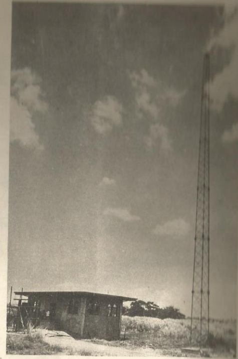
Cabanatuan Relay Station located at PAGASA Office, Cabanatuan City.
