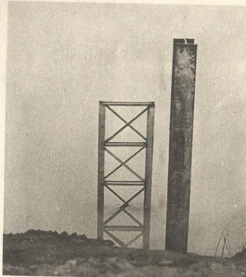
Sensing Pole Support, San Isidro Rainfall and Water Level Telemetering Station, San Isidro, Nueva Ecija.
