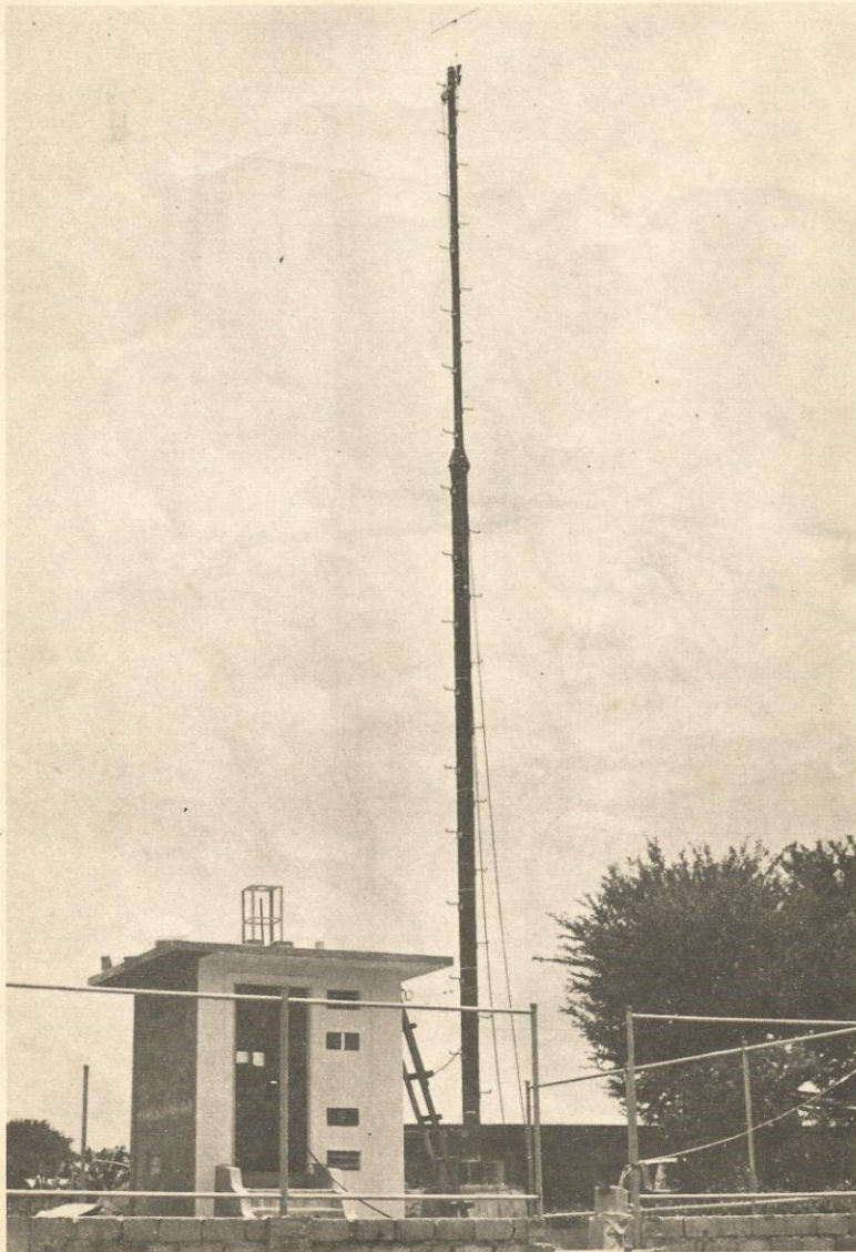
San Isidro Rainfall and Water Level Gauging Station.
