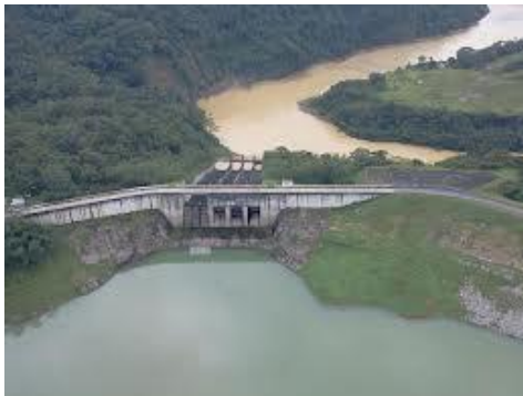
Figure: Pantabangan Dam and its spillway gates
