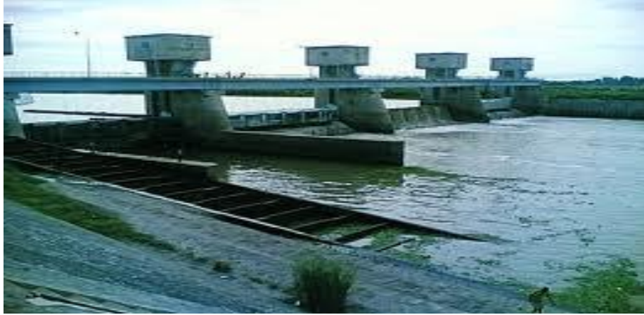
Figure: Cong Dadong Dam and its spillway gates
