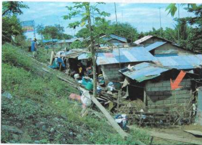
Pic 4.0 Maximum flood height (red arrow) attained as shown by the flood marks on the walls of houses that were left standing after the flashflood at the right bank of Peñaranda River (San Leonardo side).
