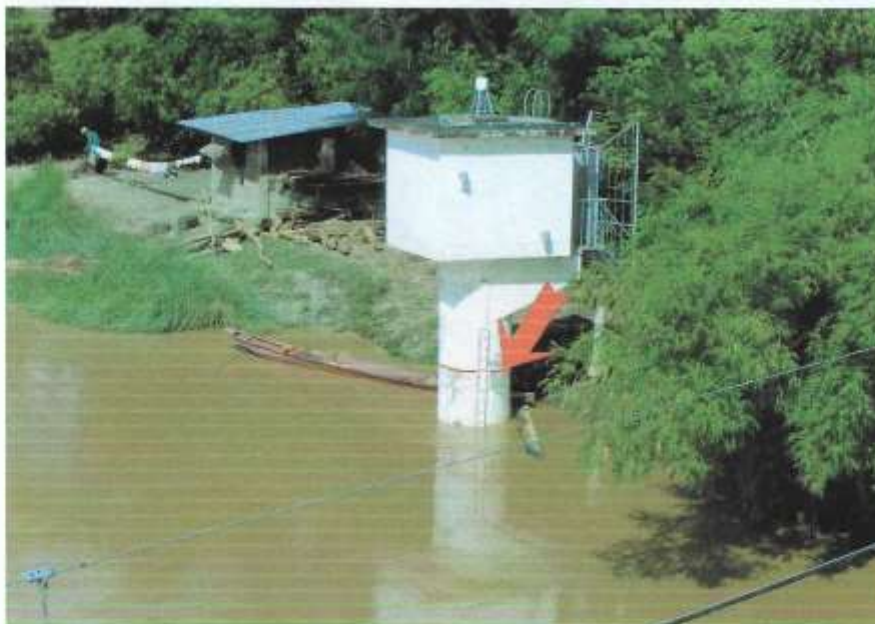
Pic 10.0 Maximum flood level attained at Arayat Gaging station reached 8.16 meters at around 1500H, 24 November 2005.
