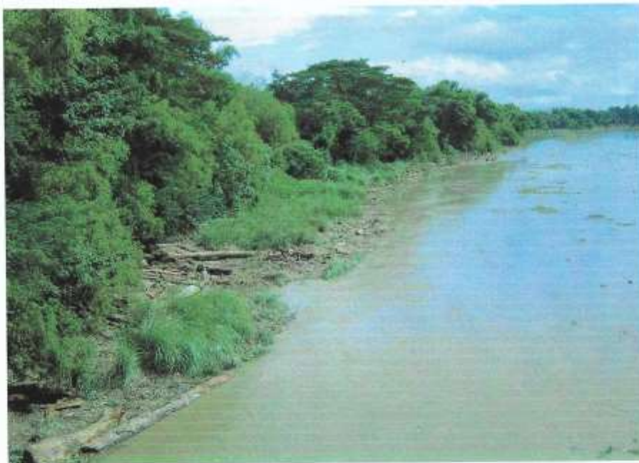
Pic 8.0 Logs that were washed away by floodwaters along the channel of Pampanga River (left bank section) at the San Leonardo-Jaen junction.
