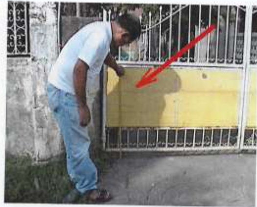
Pic 22.0 Flood marks reached 0.7 m at Bgy. San Jose, Calumpit, Bulacan.
