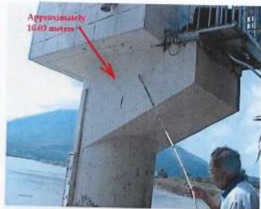
Pic 4.1 Record high of 10.03 m. registered by a flood mark attained at Arayat telemetering station.
