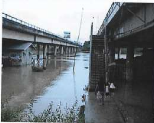
Pic 3.0 Streamgaging section in Apalit Bridge along NLEX. (August 31, 2004).
