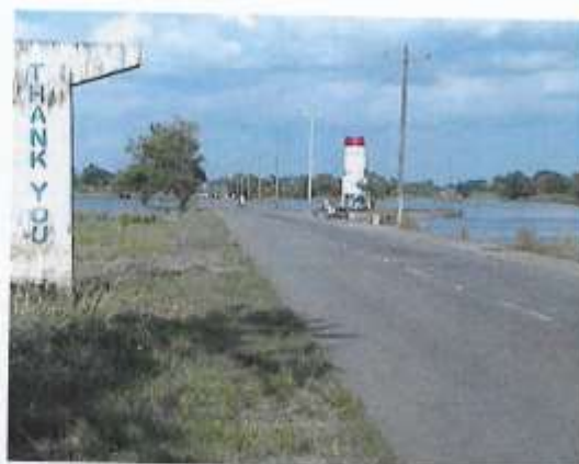
Pic 9.3 Zaragoza-La Paz Road went underwater from August 26-29, 2004 and was not passable on 27 to 28.
