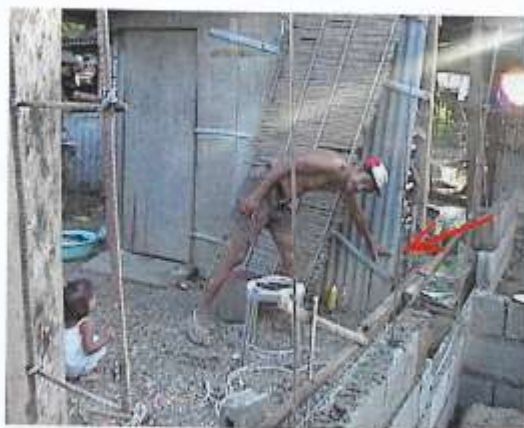
Pic 7.0 Flood depths ranging from 0.5 to 1.0 m. in Bgy. Hulo, San Antonio, N.E. (Flood peaked on August 27, 2004).
