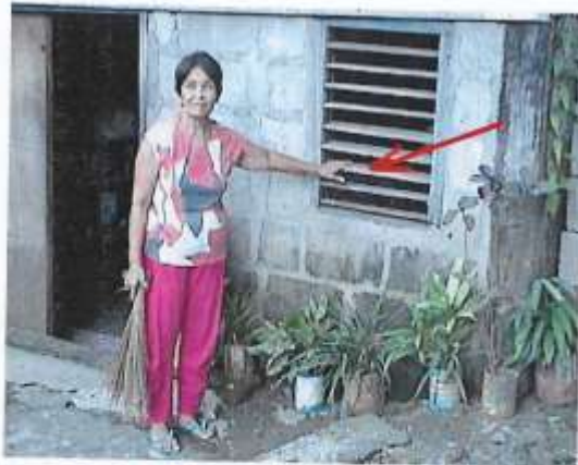
Pic. 6.0 Bgy. D.S.Garcia in Cabanatuan City underwater (August 26-27, 2004) by almost a meter of floodwaters.
