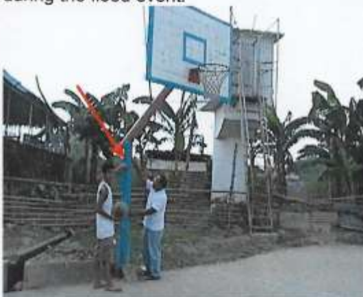
Pic 28.0 About 1.5 m of floodwaters at this part of Bgy. Sulipan in Apalit, Pampanga. Sulipan telemetering station in background.
