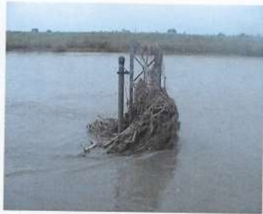
Pic 12.1 Lowest sensing pole of Sapang Buho telemetering station almost covered by debris after the flood event.
