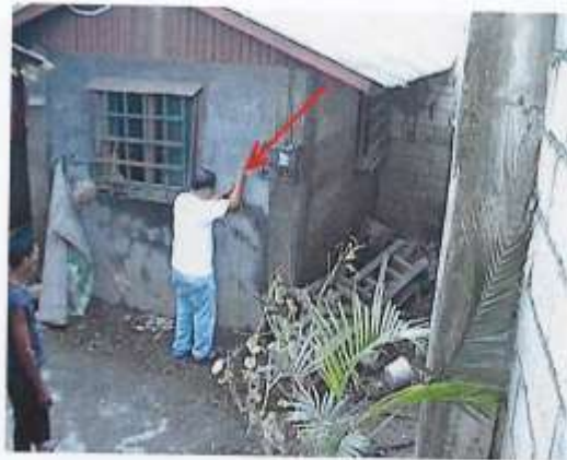
Pic 22.2 Floodwaters reached 1.4 m at Bgy. Bagbag, Calumpit, Bulacan. Peak of flooding was August 29, 2004.
