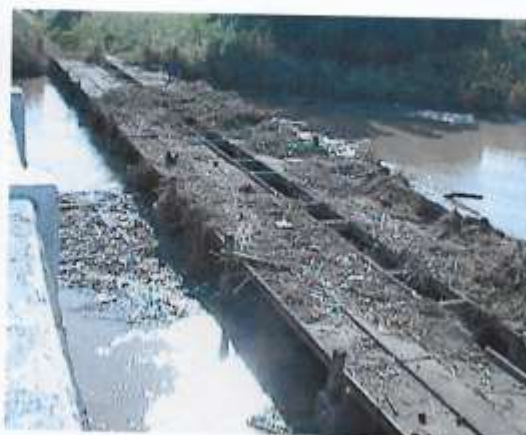
Pic 9.1 Debris strewn overflow bridge at Zaragoza streamgaging station after the flood event (September 7, 2004).
