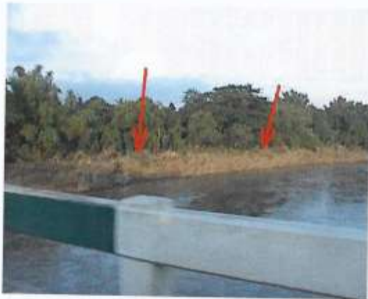
Pic 17.0 Pampanga River at San Leonardo with 2 to 3 meters flood marks at its left bank (brown foliage).
