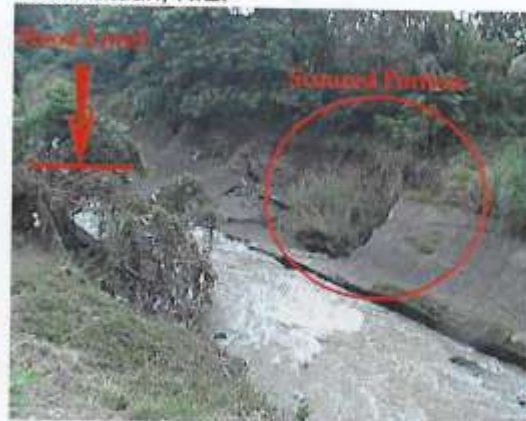
Pic 8.0 No overflowing of Minatula River (Cabanatuan) during the event but flood flows scoured portions of the river dike.
