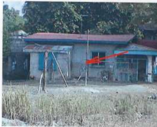
Pic 22.8 The same house / area above this photo (Pic 22.6) a week after the event (taken September 9, 2004).
