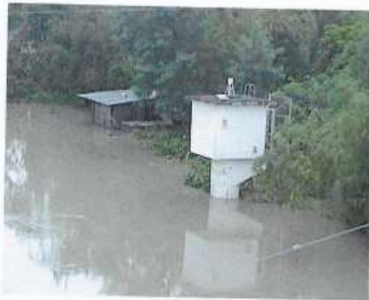
Pic. 4.0 Arayat telemetering station at stage 8.65 m., 4 days after its recorded peak stage of 10.03 m.
