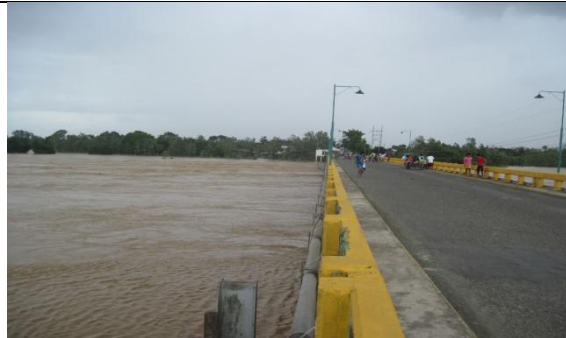
Downstream, RB view (station side) of the Pampanga River at San Isidro station at a S.G. reading of 7.4 meters (estimated)
