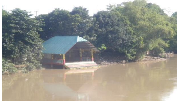
Pampanga River at NLEX-Apalit Bridge; Sulipan S.G. reading at 2.25 meters (estimated); Boat ferry landing platform starts to get flooded between S.G. of 2.65-2.85 meters (estimated) at Sulipan stn.
