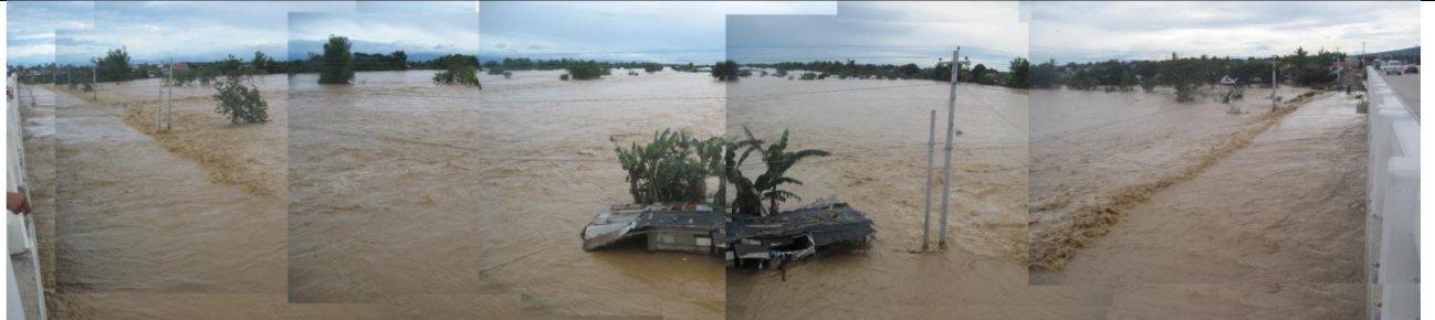
The Cabiao Floodway situation at an Arayat S.G. reading of 9.6 meters (estimated); Cabiao Floodway gets overflowed at an estimated Arayat S.G. reading of 8.6-8.8 meters (still for validation).
