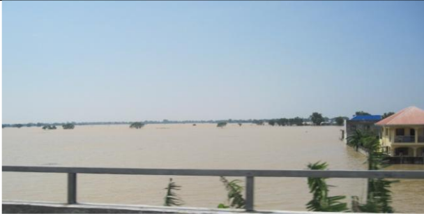
Flooding at lower Candaba area along NLEX-Viaduct at a Candaba telemetry reading of 7.07 m & Sulipan telemetry reading of 4.19 m (or S.G. reading of 4.33 m., estimated); Candaba had already peaked 5-6 hrs before & higher by 0.06 meters only.
