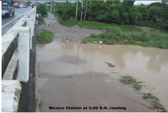
Mexico station: River has already overflowed the old bridge's floor at upstream of the station at a telemetry reading of 0.90 m.
