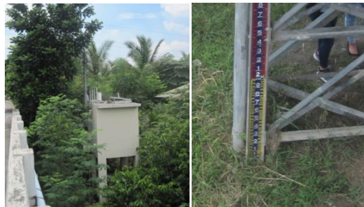
The latest situation of the station housing, the S.G. and sensor which is about a meter below the ground
