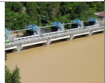
Ipo Dam reservoir
