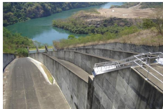
View of the Pantabangan Dam spillway
