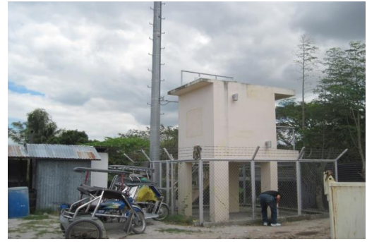
The Porac RR telemetry station
