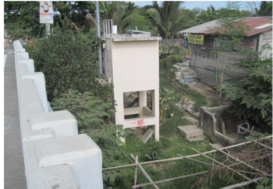
The station as seen from the Mexico Bridge No. 2
