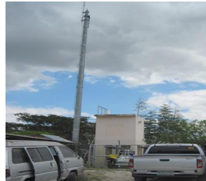
Another view of the Porac RR telemetry station
