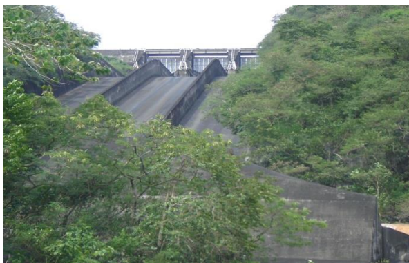
View of Angat Dam spillway
