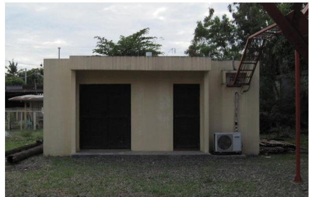
The RR and repeater station housing
