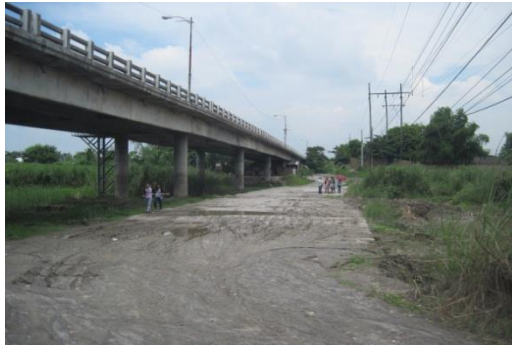
The old overflow bridge at upstream of the Mexico Bridge No.2 is shown above.
