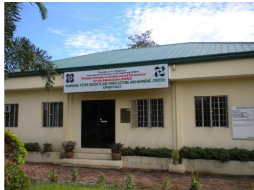
The operations building of the PRFFWC in CSFP, Pampanga (Inaugurated March 2009)
