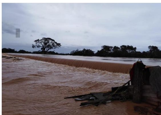
Figure 7.9 (top L) Overflowing Creek going to Maasim River at Bgy. Maasim, San Rafael, Bulacan taken at around 0500H-0600H of Nov 12; floodwaters started around 0300H to 0400H of Nov 12 and totally subsided before midday of the same day; overflowed waters reached from 1.0 to 1.5 meters above the road. (top R) Same creek during normal flow situations. (pictures provided by Mr. L. Rodriguez)
