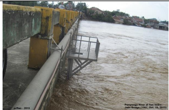
Pampanga River at San Isidro-Jaen Bridge at a gauge reading of about 7.60 meters (1307H, Oct. 19, 2015); Pampanga River was already in recession phase at this time; at the background are riverside houses that are still partly flooded by the river.
