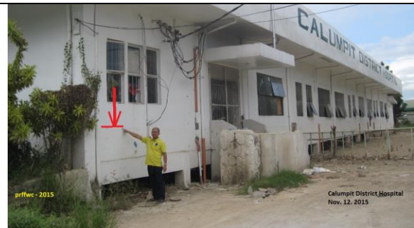
Maximum flood height reached at the Calumpit District Hospital reached to more than 1.5 meters from ground level. Note that hospital is already elevated by several centimeters from the ground. (Nov. 12, 2015)
