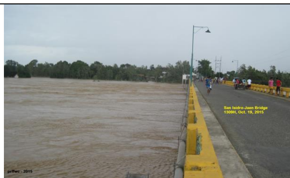
(Top left) The Pampanga River at the San Isidro-Jaen Bridge at a relatively low river stage below the "0" gauge reading of the San Isidro telemetry station (Dec. 09, 2015); (Top right) The same spot during event Lando at a telemetry gauge reading of around 7.60 meters (1309H, Oct. 19, 2015).
