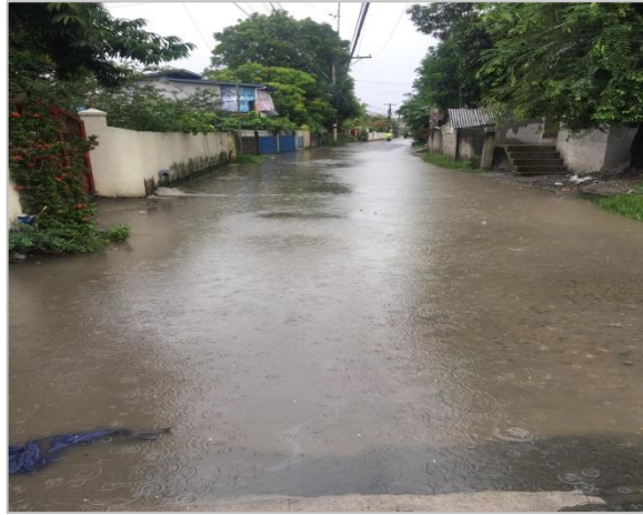
Photo 4: No drainage/canal systems
