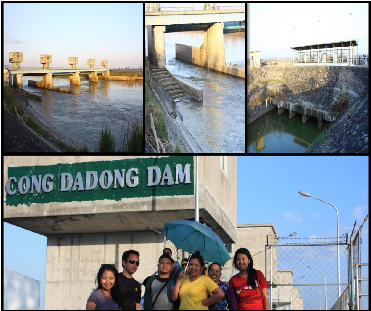
Figure 10. The Cong Dadong Dam
