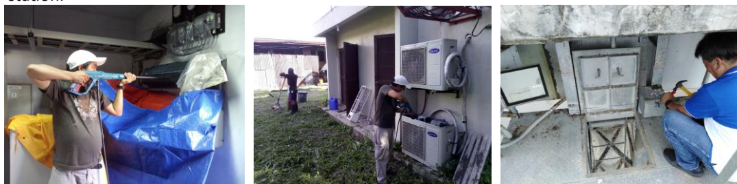
(Above pictures, Left & Middle) Cleaning of air conditioners at San Rafael Repeater station; (Right) PRFFWC personnel supported HMTS in the replacement of WL sensor at Zaragoza station (August 23, 2019)
